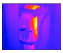
Figure 5: Damaged breaker contacts can cause resistive heating. Thermal patterns from these poor connections appear as diffuse heating on the surface of the breaker.
