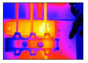
The bus stabs and the connections to the main are important inspection points that are often overlooked or misdiagnosed. The incoming connection to the main horizontal bus is usually located behind a cover or panel that is not hinged. These are typically bolted connections and may have parallel feeders.
